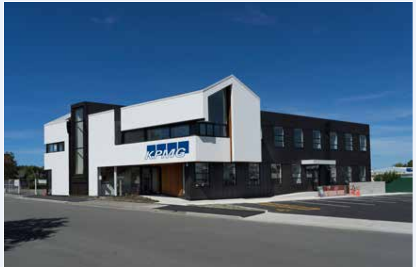
KPMG Timaru's new premises The Terrace
